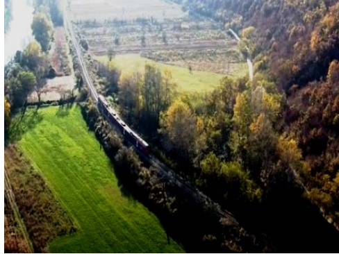
Existing railway track, line Stalać – Djunis, by river Južna Morava
