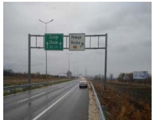
Insufficient distance of gantry pillars from carriageway edges
