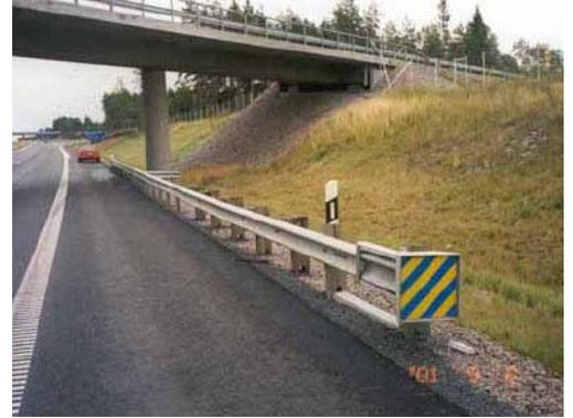
Example of a correctly placed and absorbent crash barrier at a structure.
